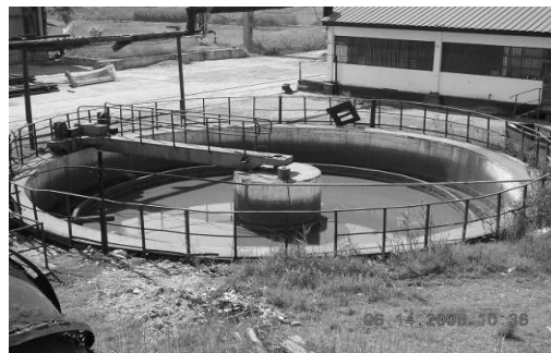
Fig. 2 Centrifugal settling tank
