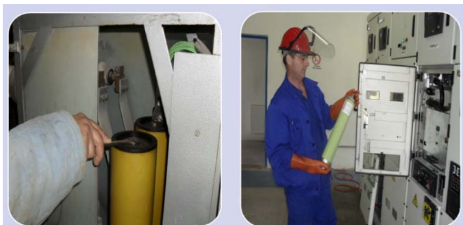
Fig. 14 – Cells' fuses II.
