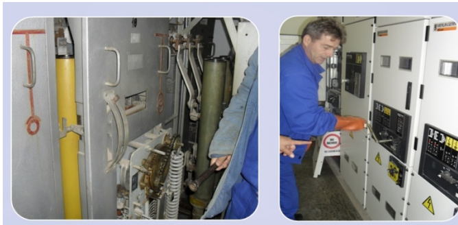
Fig. 4 – Opening the cell's door II.
