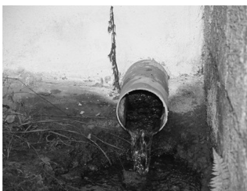
Fig. 1 – AMD drainage pipe - sampling point.
