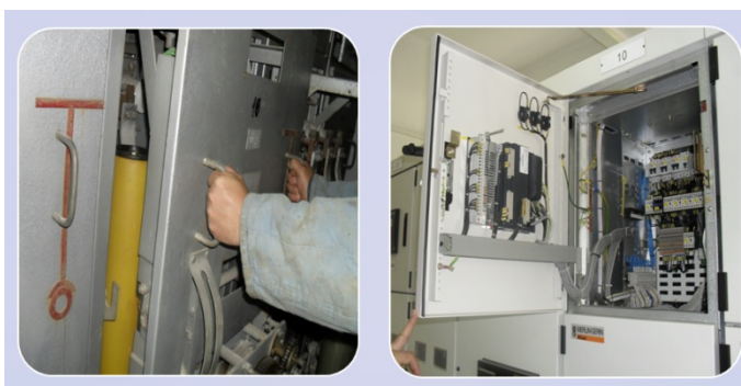
Fig. 13 – Cells' fuses.
