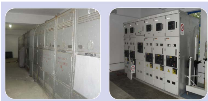
Fig. 2 – Access to cells: Old station - access possible via backside and frontside. New station - access possible only from frontside.
