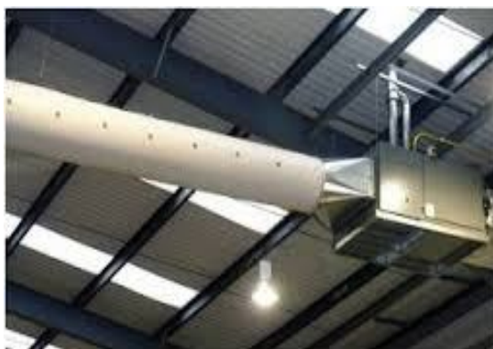
Fig. 3 – The installation of noxes ventilation system.
