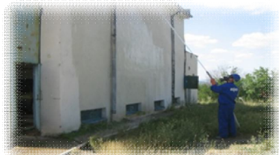
Water curtain made by worker (old facility)
