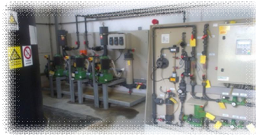
Modern chlorine dosing plants
