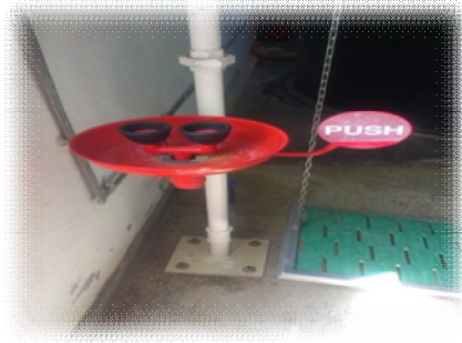
Special eye washing device in new facility
