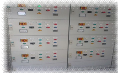
Modern electric panel
