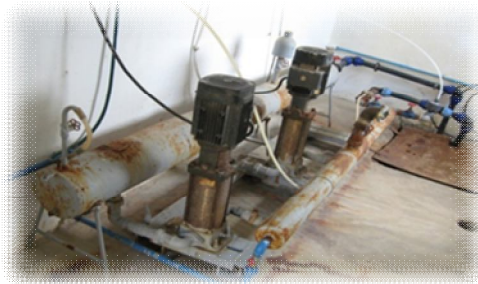
Improvised chlorine dosing devices (risk of chlorine poisoning)
