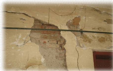
Plasterings damaged by reagents
